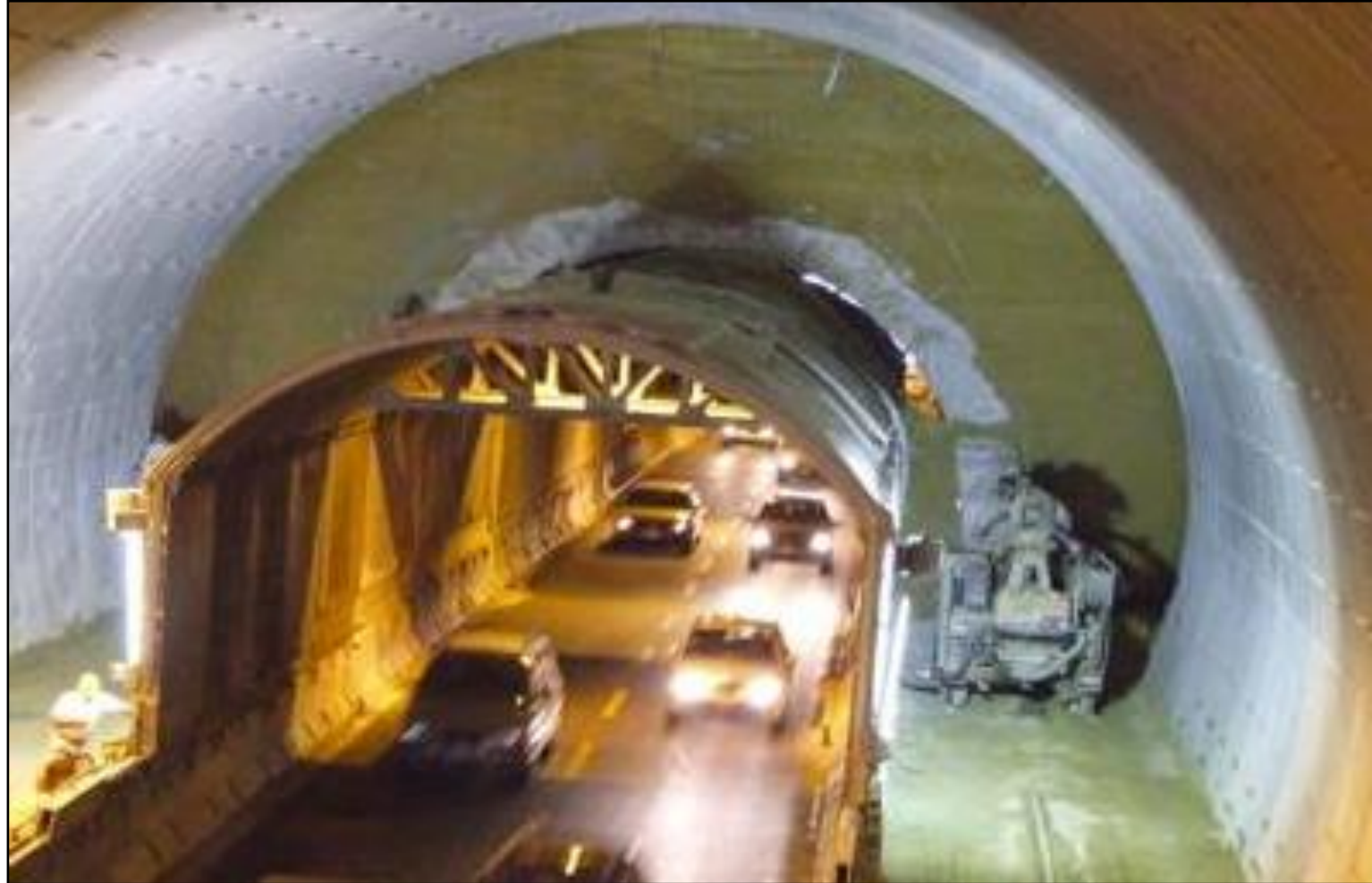
Nazzano Tunnel (Highway A1) - with vehicular traffic during work
