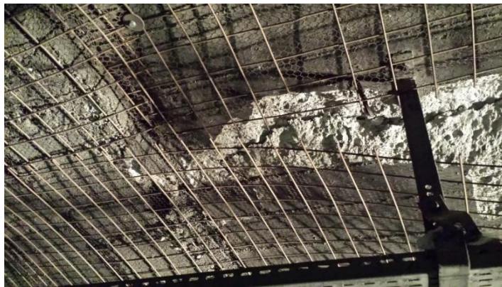
Vault concrete detachments
