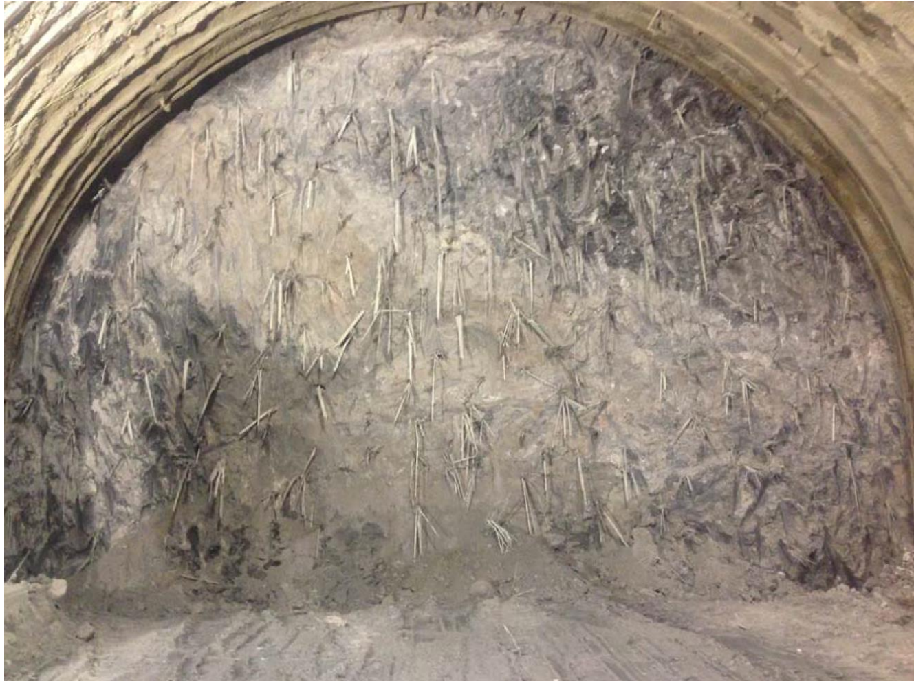
Siena side - face immediately after the excavation restart (formation: GP/CV )
